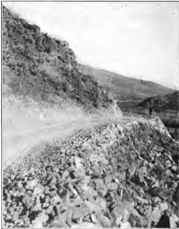
State Road Through Circleville Canyon, Garfield County, Showing Sidehill Construction.
